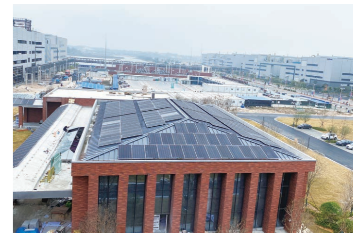
PV Equipment Site at Qinzhou Industrial Base
